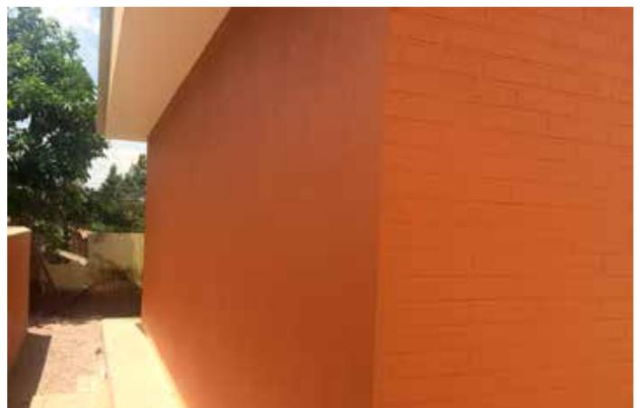
*Coating with brickwork effect*
