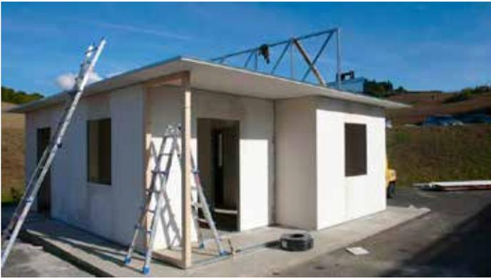
*The false ceiling/eaves system and the steel truss system*
